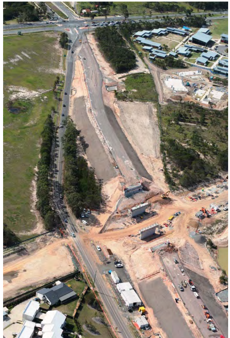
Bridge progress looking north towards Anzac Avenue
